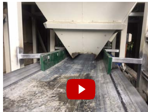
LEFT Image AFTER Installation
