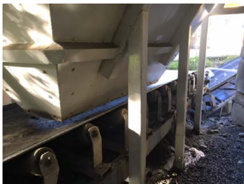
RIGHT Image BEFORE Installation
