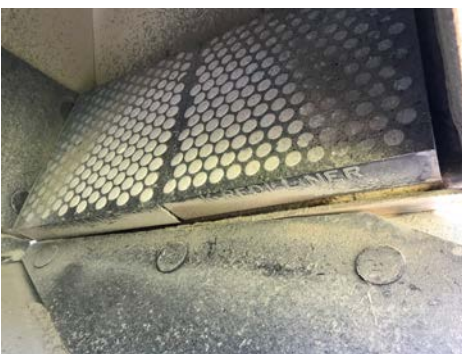
LEFT K-Redi-Liner® Ceramic Installation
